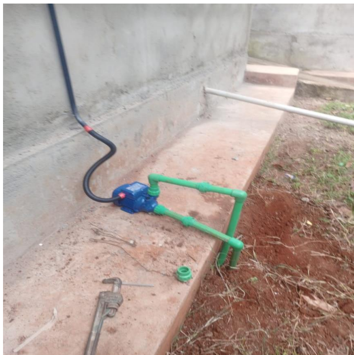
A pump for pumping water in the upper tank
