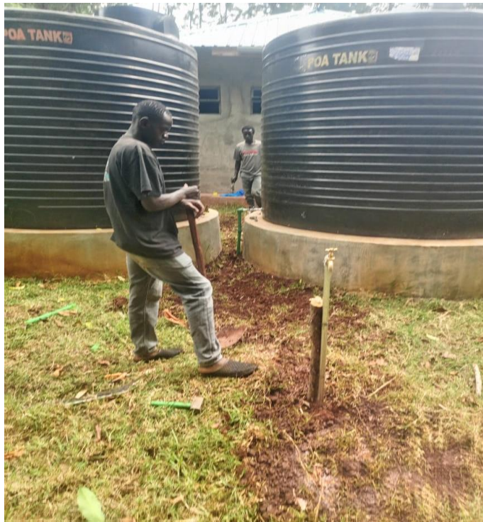
two tanks 10,000 liters each for harvesting water from the roof
