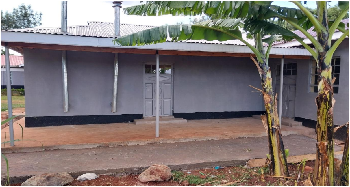
Rear view completed kitchen
