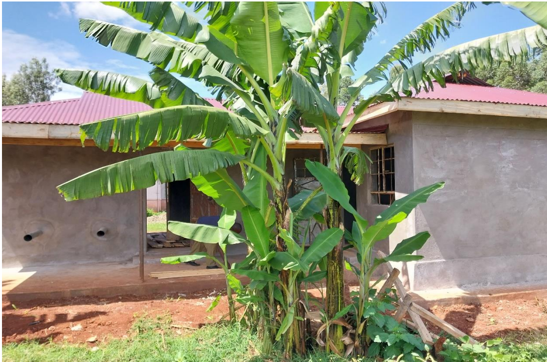
Rear view , plasta done, chimney fixed , faciaboard fixed
