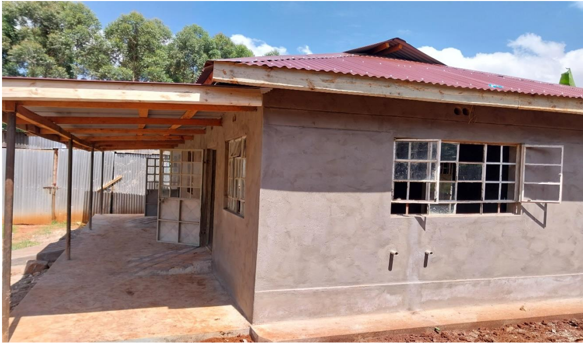
Side view of the kitchen
