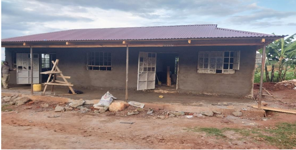
Front view of the kitchen. Plasta already done
