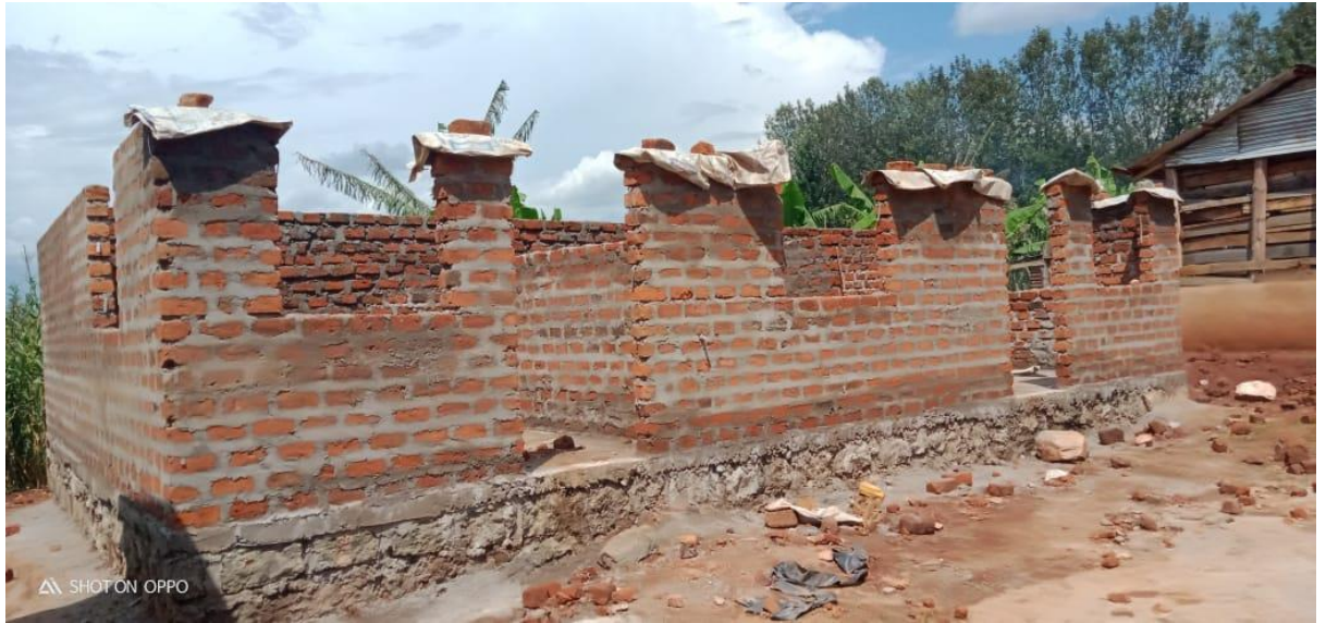
Good progress of construction
