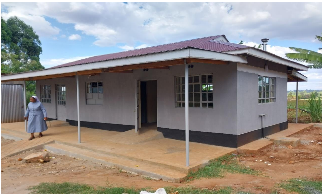
Front view, completed kitchen
